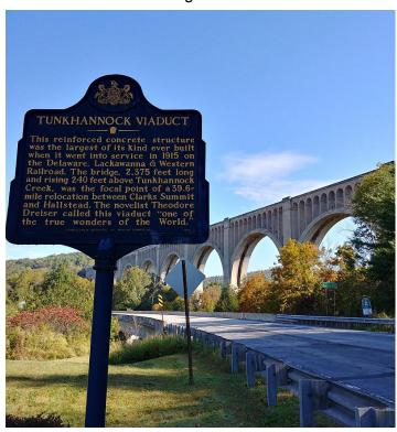
The Tunkhannock Viaduct is located in Nicholson, PA. Construction was finished in 1915. The bridge is 2375 feet long, 34 feet wide, and 300 feet high at it's tallest. At the time it was constructed, it was the largest concrete structure in the world.
