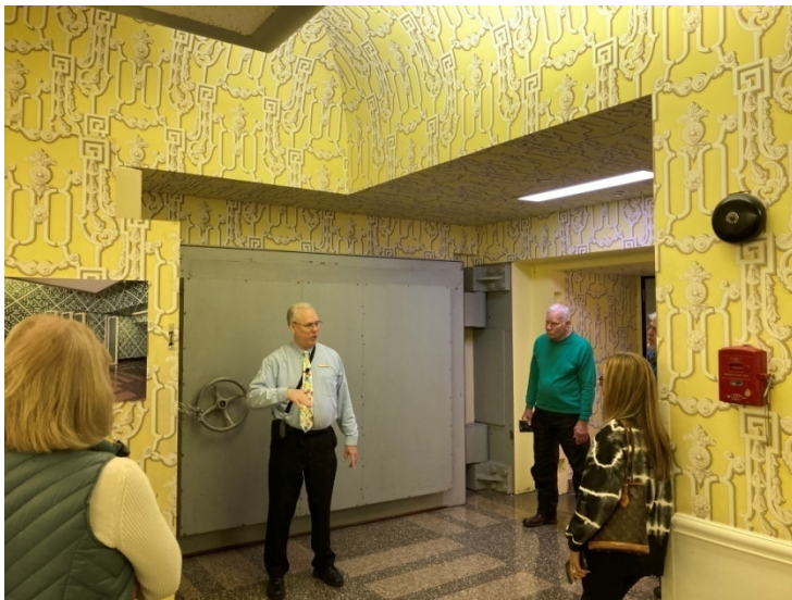
Greenbrier Resorts BUNKER entrance. Door is 2 feet thick. Entire bunker is encased in 5 feet reinforced concrete. Huge 112K sq ft. 2 story bunker. It was built to withstand an atomic hit. Check out the door knob and door hinges. It was capable of holding 1100 Congressional occupants for several months.
