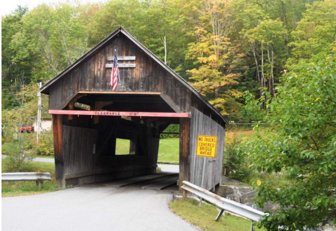
Vermont is noted for covered bridges. This one was in the very small town of Warren.
